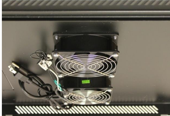
Cabinets Fans for Ventilation
